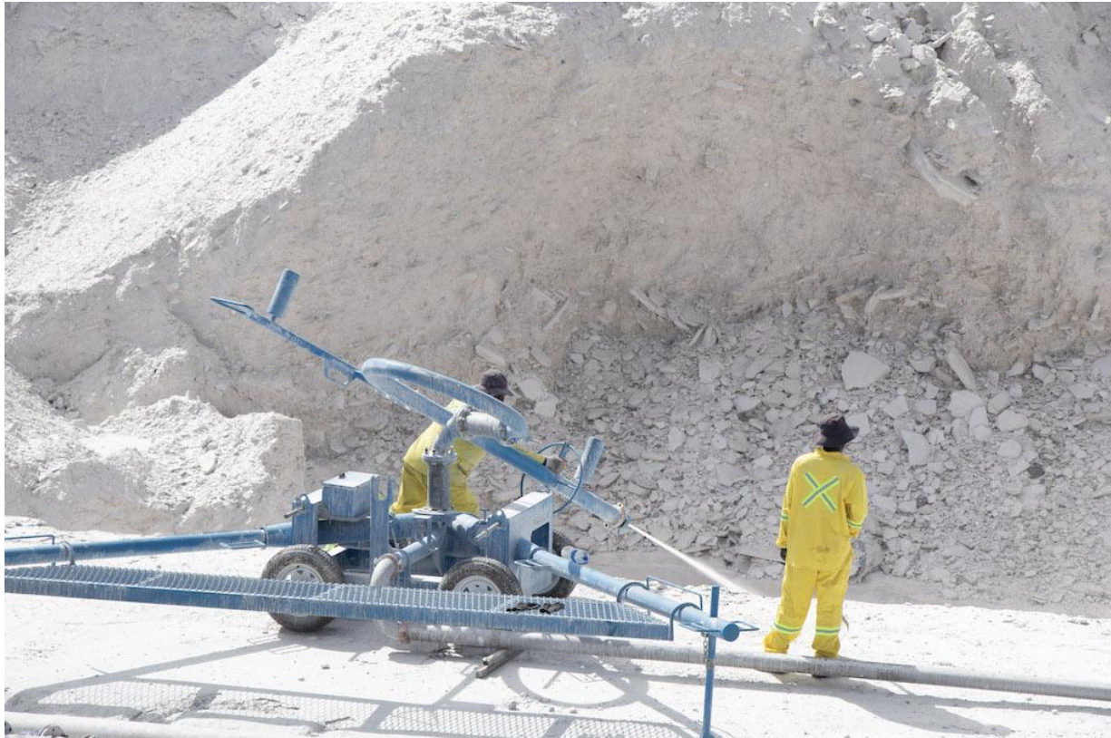
Contractors from Paragon Tailings doing trial hydraulic reclamation of the phosphogypsum stacks. Photo supplied
